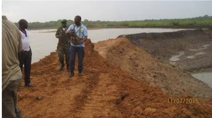
Dam in a creek under construction
