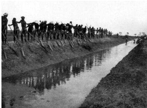
Traditional construction of a Bolanha dike and drain by Balantas
