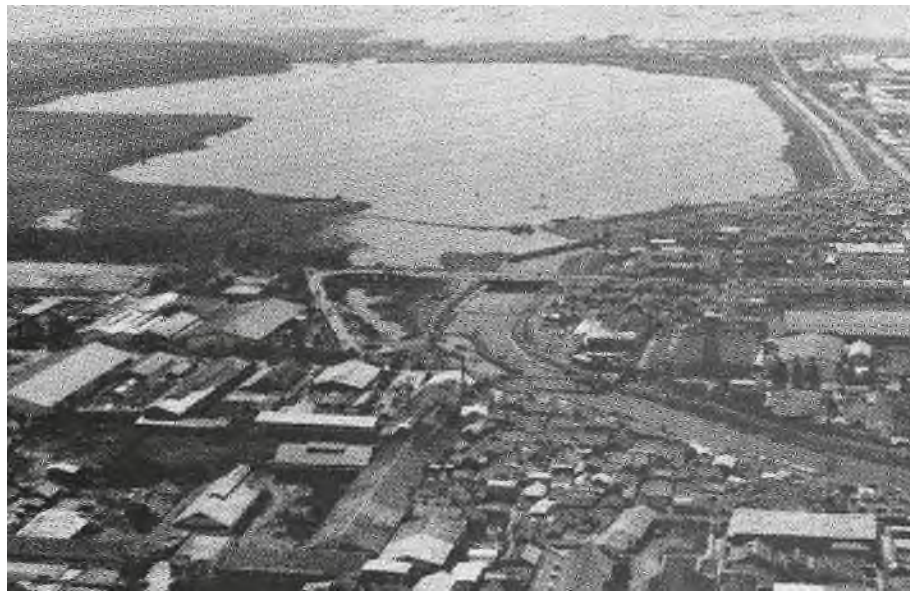
Figure 2. Aerial view of the storage reservoir and waterworks in the Pluit Polder (Kop et al. , 1983)
